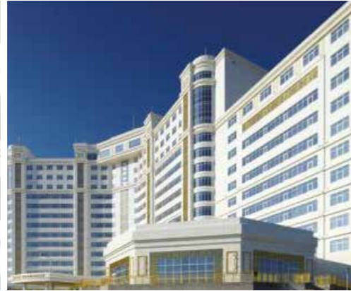
VIP Otel / Türkmenistan
